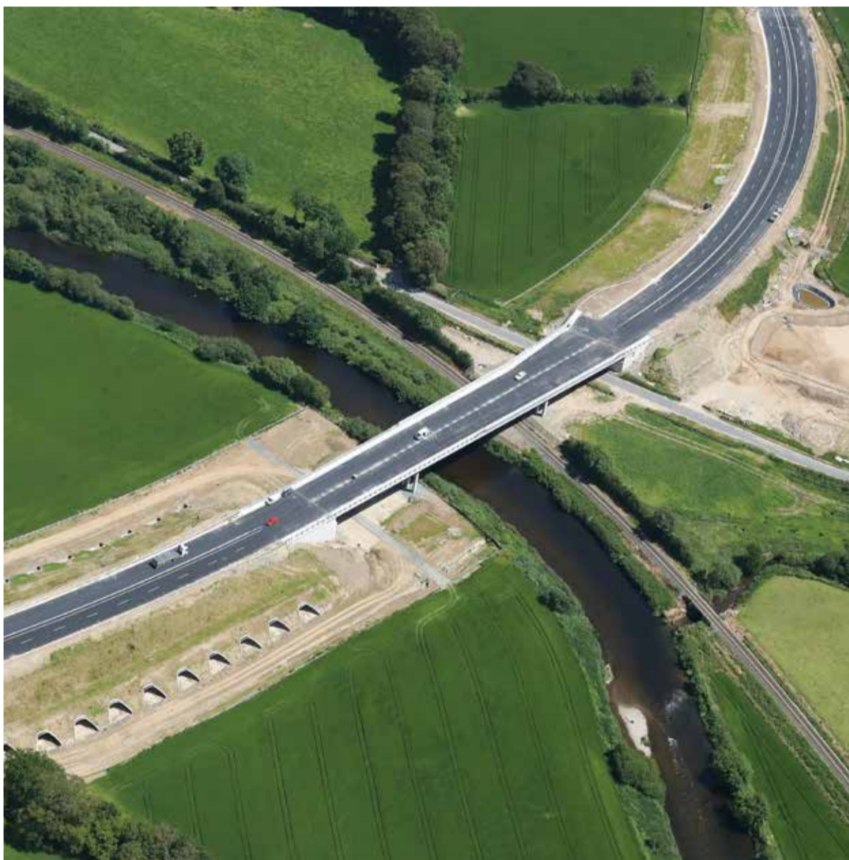
River Slaney Bridge M11, Gorey to Enniscorthy PPP Scheme
