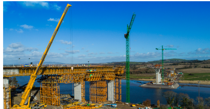
N25 New Ross Bypass River Barrow 3 tower extrados bridge construction
