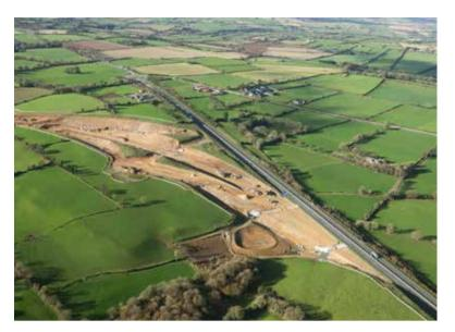
The majority of the works that are weather dependent have been substantially completed, like earthworks and stream diversions, which allow our teams to focus now on drainage works, pavement works on M11, N30 and the N80
