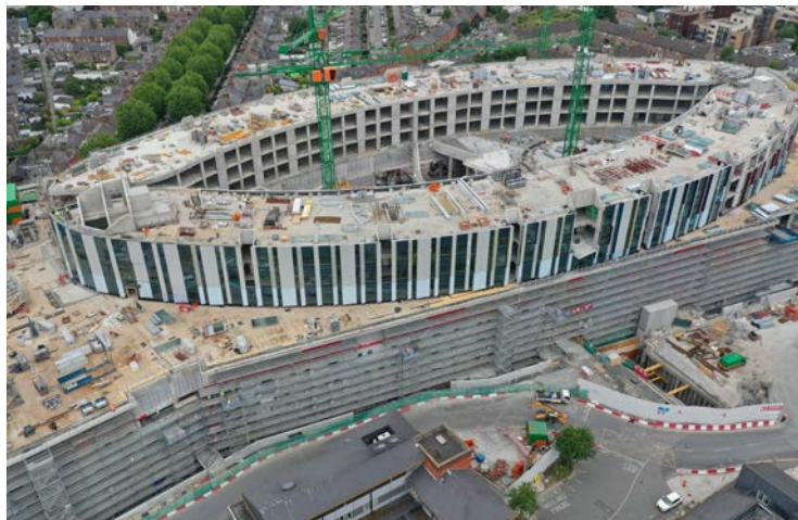
New Children's Hospital under construction
