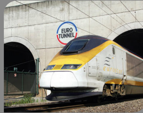
2 The Channel Tunnel, completed in 1994, connects Great Britain to Europe through three, 50km long tunnels. 37km of this tunnel are underwater.
