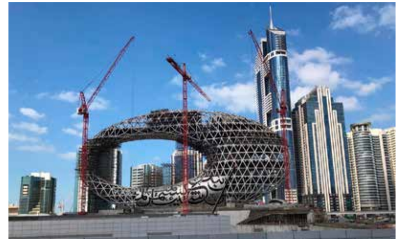
Museum of the Future under construction
