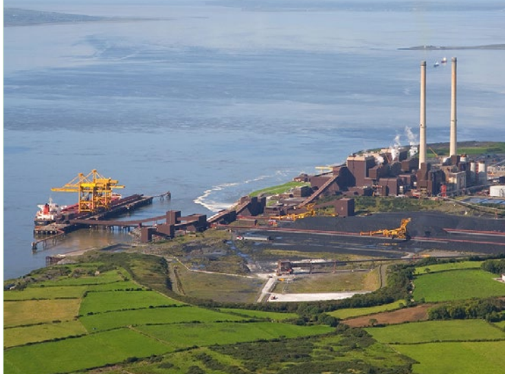
BAM Ireland completed Moneypoint Power Station in County Clare, Ireland's second largest power station, in 1985.
